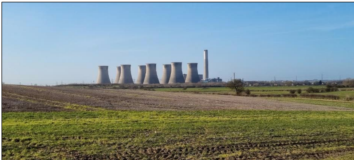
Plate 36: View southwest from the Viking Winter Camp towards Cottam Power Station
