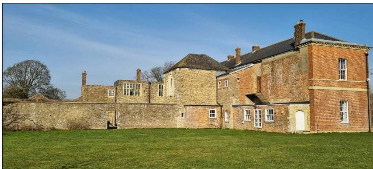
Plate 28: View of the rear elevation of Glentworth Hall
