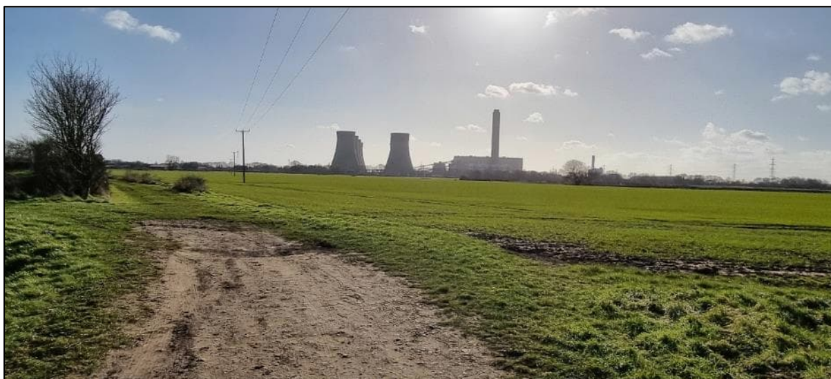
Plate 43: View south across the Cable Route Corridor towards Cottam Power Station
