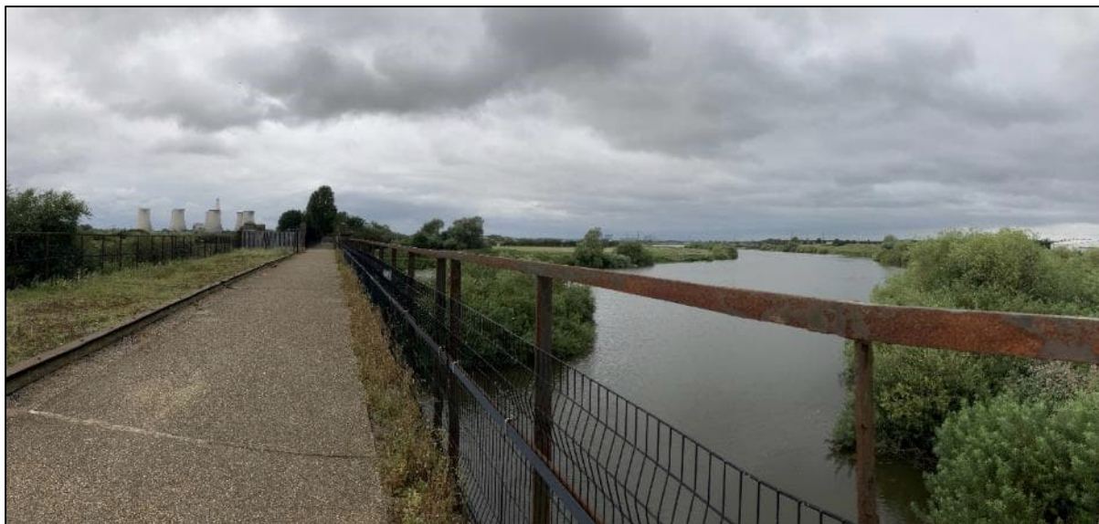
Plate 40: Panorama View from the viaduct looking northwards across the River Trent
